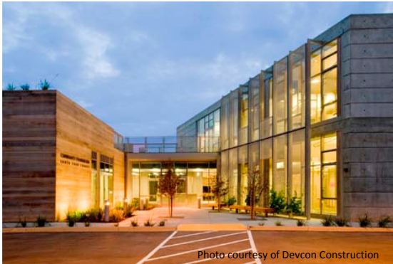
Photo courtesy of Devcon Construction
