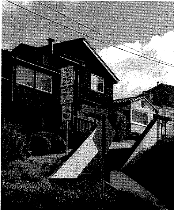
Smooth Finish Concrete Retaining Walls to Match Existing Nearby Stairs
