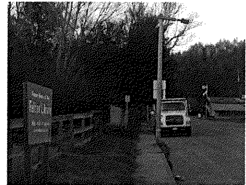
Figure 8 – Existing wooden streetlight pole near driveway for proposed Felton library.
