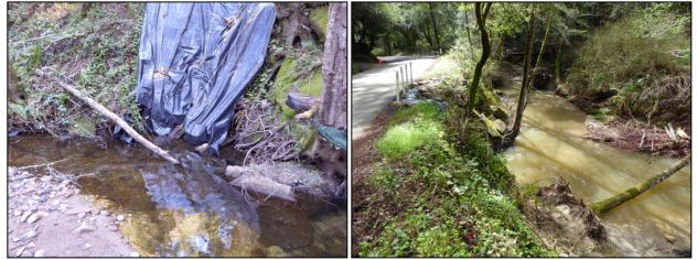
LEFT: Eroded left bank and scour pool at toe of slope. RIGHT: Project site looking downstream after early March 2016 high flows.
