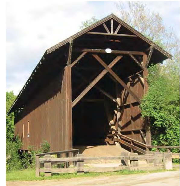
Felton Covered Bridge County Park
