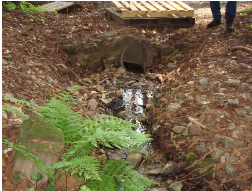
Figure 7. View of Intermittent Creek and Concrete Culvert, April 2022
