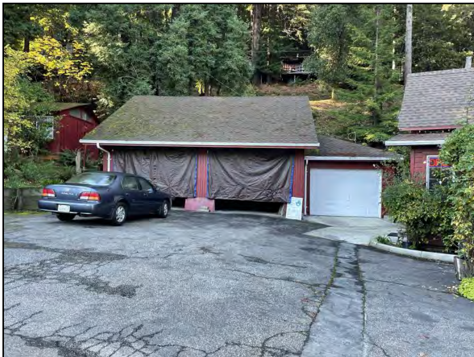
4 : Main residence garage.
