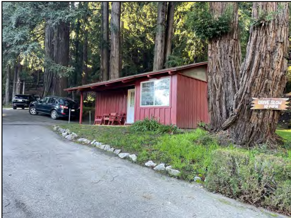
6 : View of access road near cabin #5.
