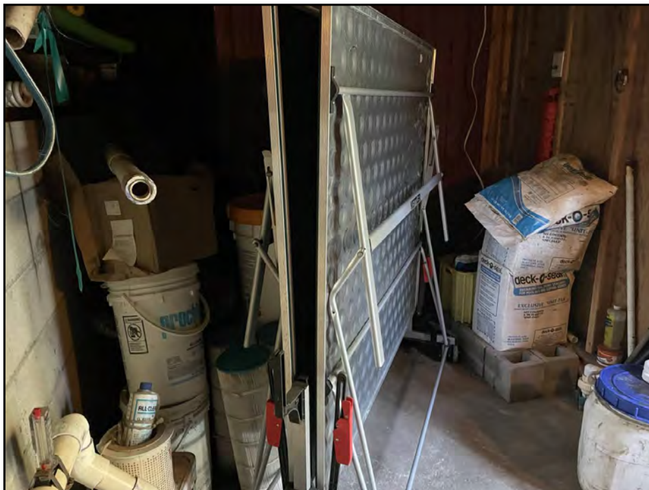
28 : Pool chemicals stored in structure adjacent to pool.
