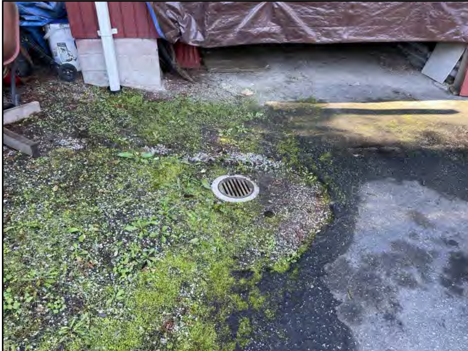
31 : Storm drain adjacent to residence garage.
