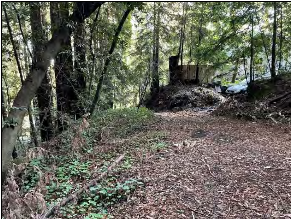
24 : Unimproved access road in southern portion of Property.
