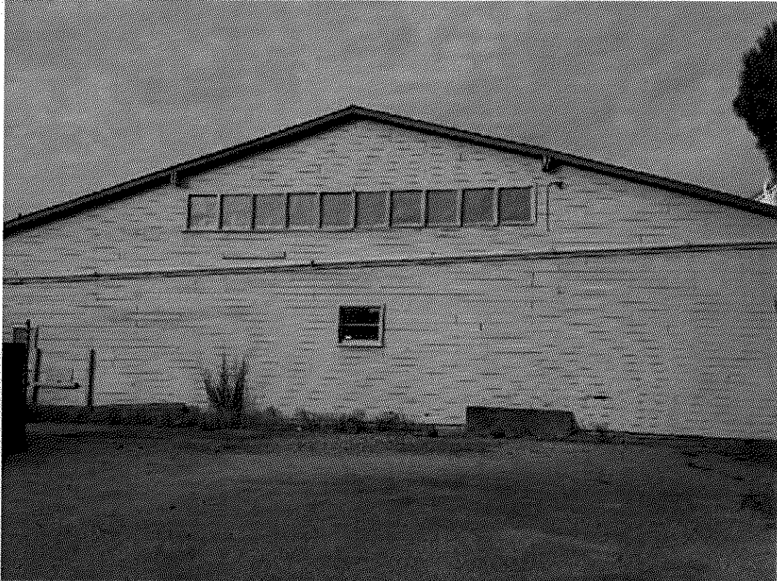
BUILDING SOUTH SIDE VIEWED FROM SOUTHEAST PROPERTY CORNER
