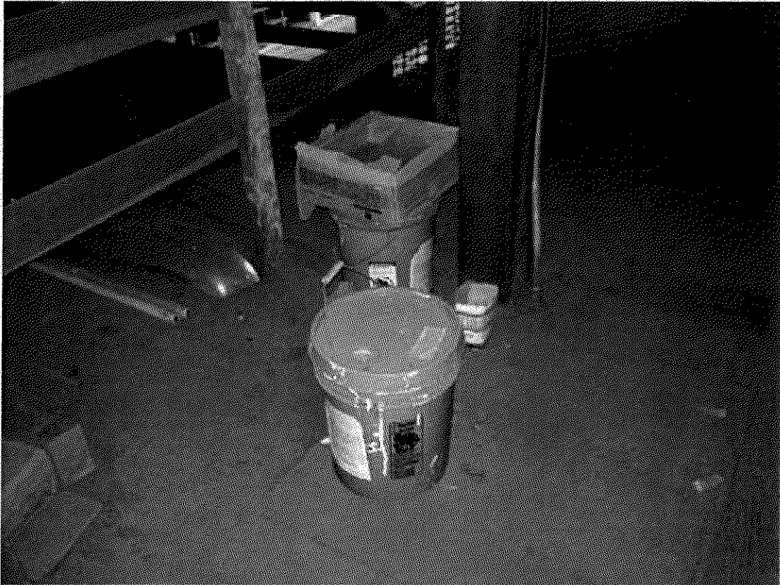
PAINT BUCKETS STORED ON MEZZANINE LEVEL
