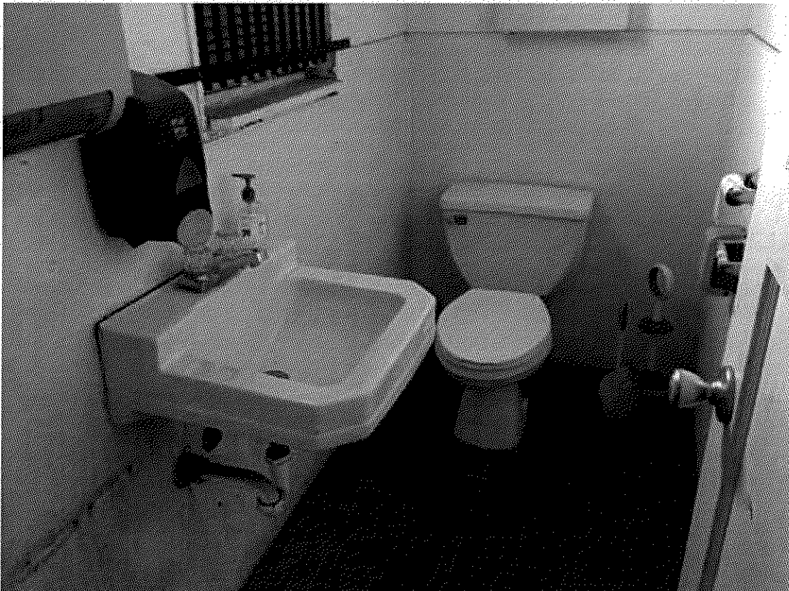
RESTROOM IN SOUTHWEST CORNER OF BUILDING
