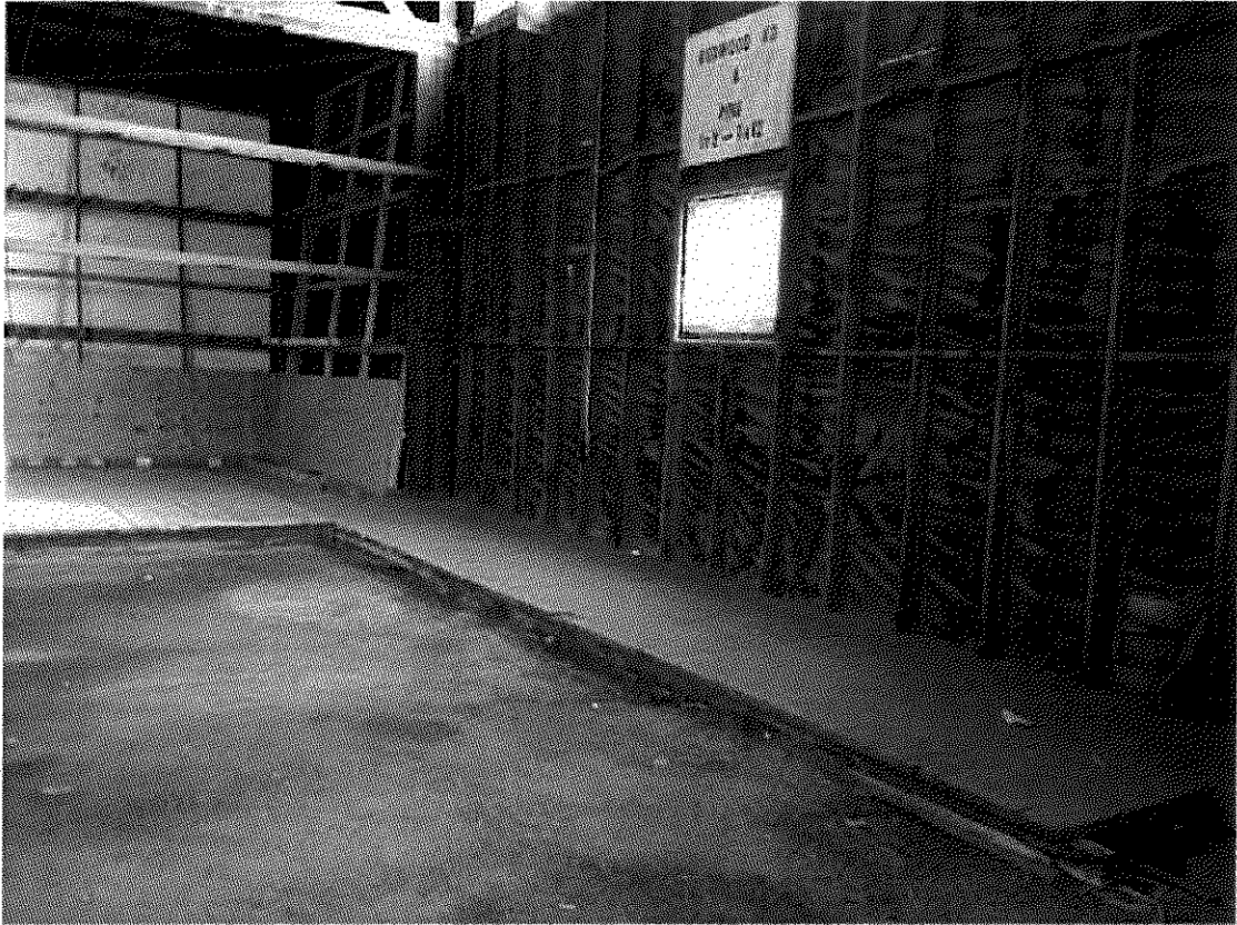
BUILDING INTERIOR, SOUTHWEST CORNER
