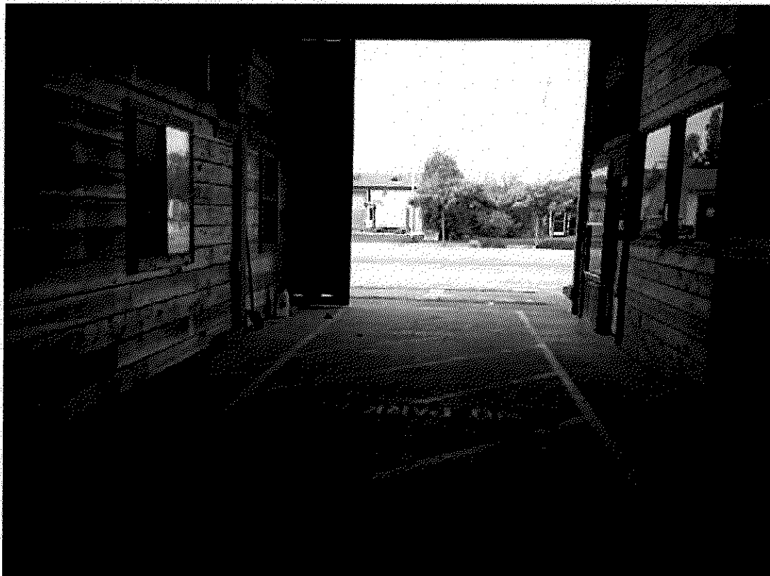
BUILDING ENTRANCE ON NORTH SIDE, VIEWED TOWARD PORTOLA DRIVE
