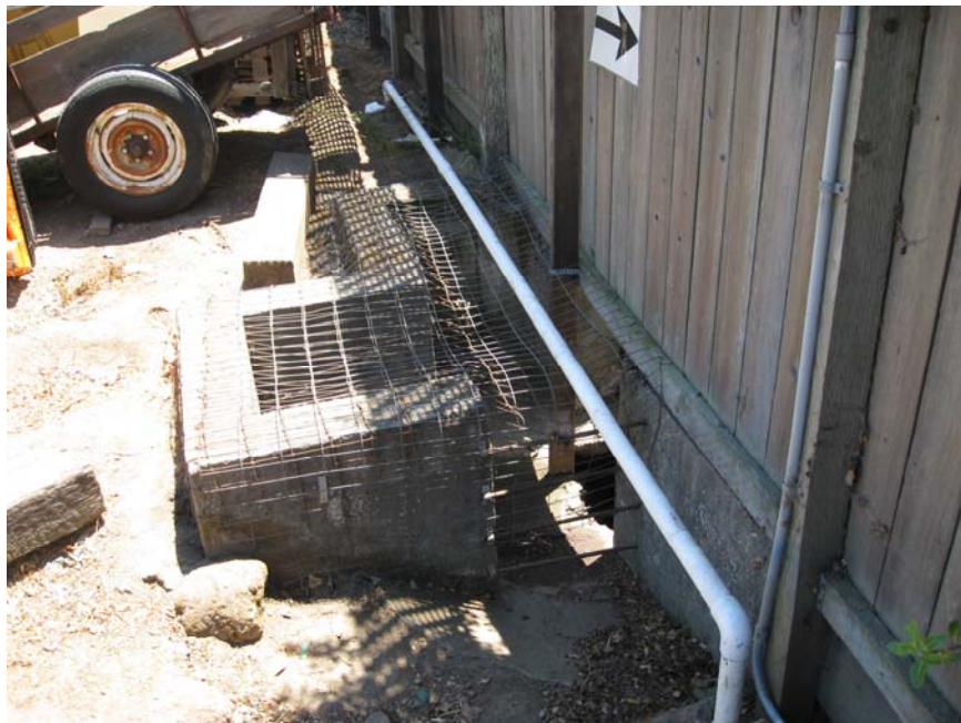
Concrete headwall outlet structure
