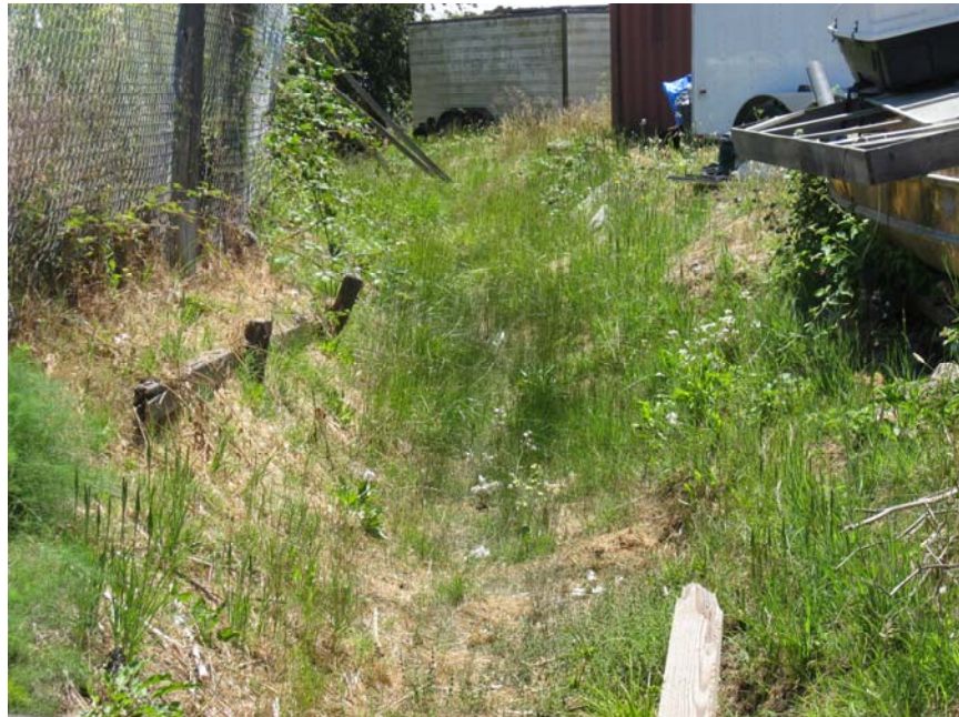
Looking downstream at vegetated swale
