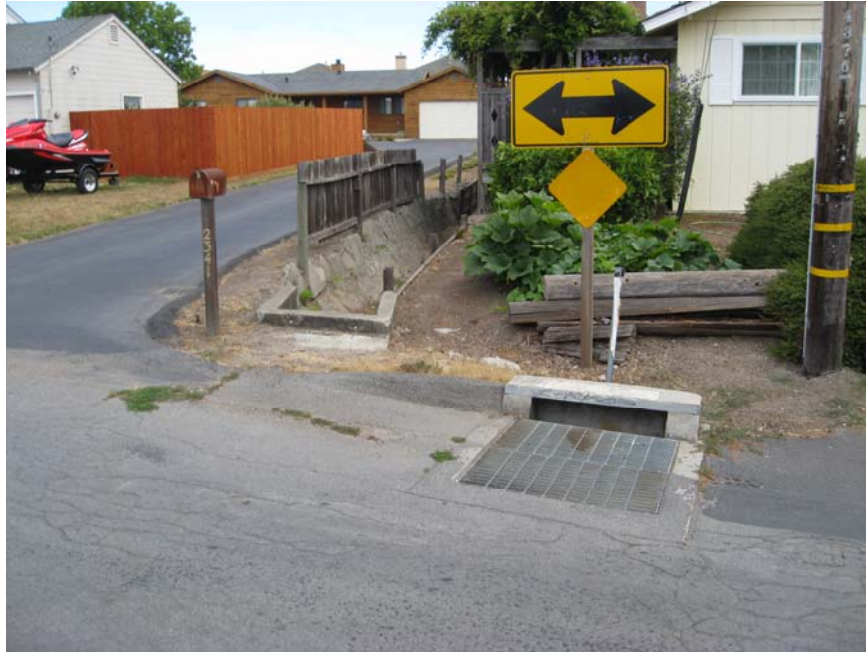
Curb inlet along Mattison Lane
