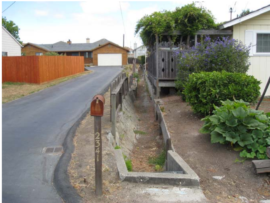
Open concrete channel and inlet along Mattison Lane
