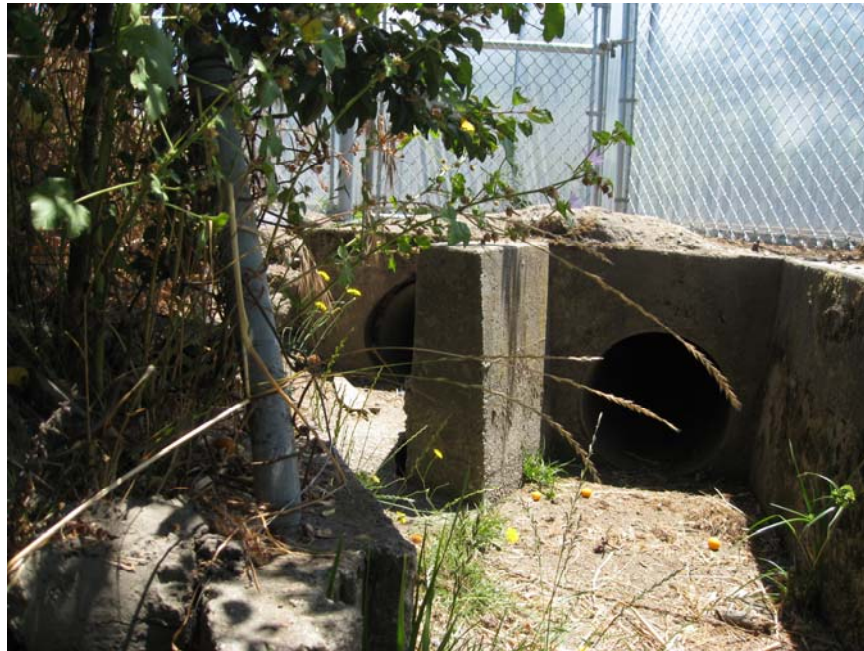
Concrete headwall with 18" RCP inlets
