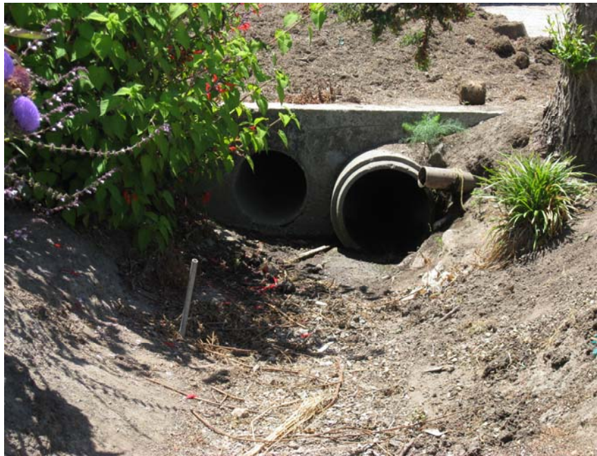
Concrete headwall and inlets in graded swale
