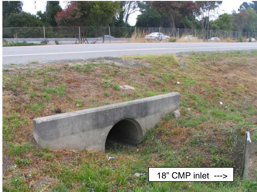
Concrete headwall with 36" RCP outlet and 18" CMP inlet
