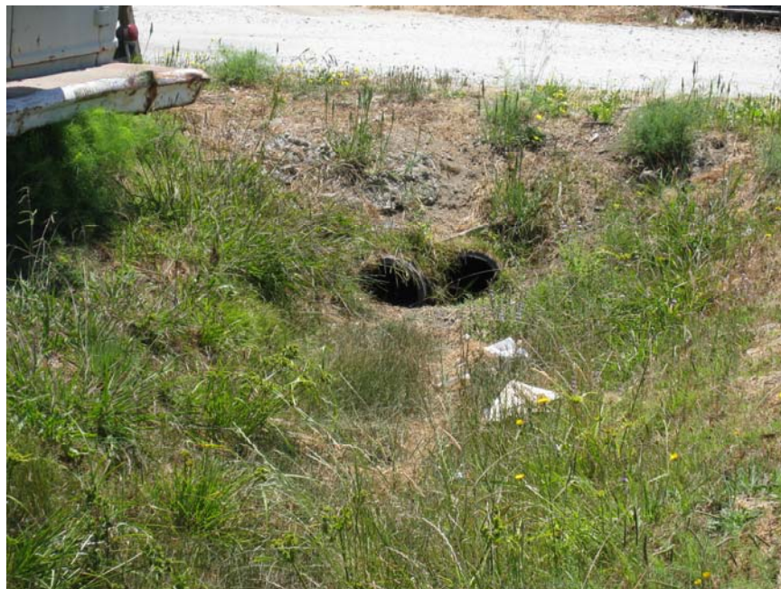
Dual 12" HDPE inlet pipes in vegetated swale
