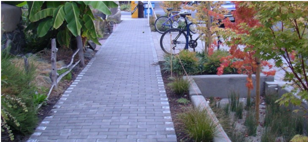
Permeable paving and landscaping capture and percolate stormwater runoff Photo Credit: MIG, Inc.
