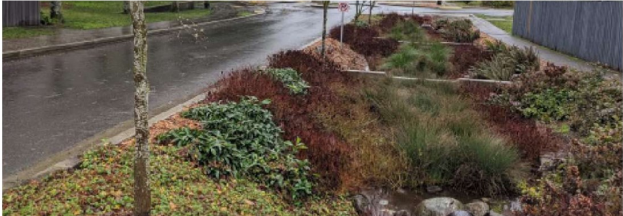
Bioswale collects and filters stormwater
