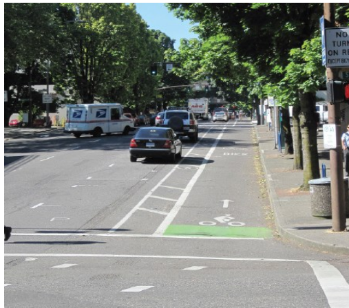
Buffered bike lane. Photo credit: Fehr & Peers, 2014
