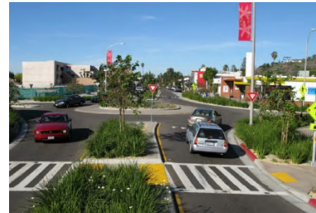
Pedestrian refuge islands provide a protected resting place for pedestrians when crossing wider streets – approximately more than two lanes of traffic. Photo Credit: Model Design Manuel, 2010.
