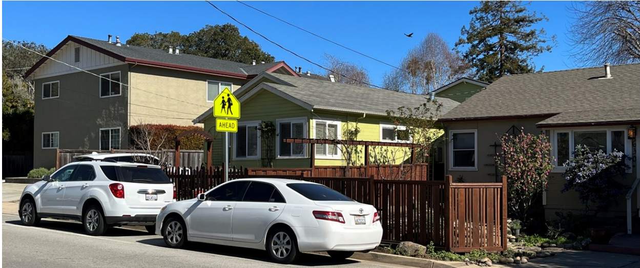
Live Oak Neighborhood with mix of apartments, small-lot single family dwellings with ADUs, and condominiums. Photo Credit: Santa Cruz County.
