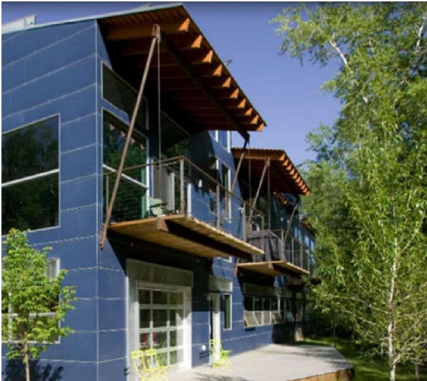
New and existing trees buffer adjacent development.
