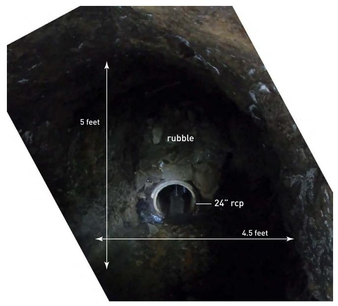
Drainage Tunnel B at Reinforced Concrete Pipe - view is downstream.
