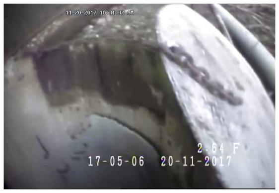
Photograph 4: Exterior view of the western shaft with lid at transition to Highway 1 culvert.
